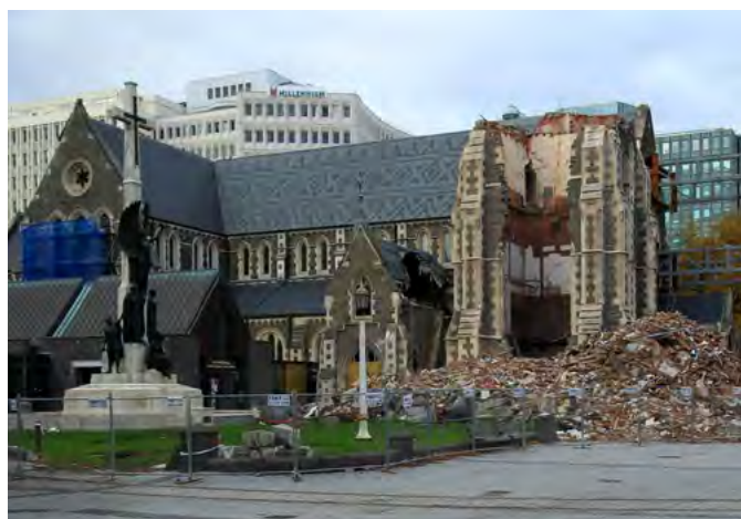
NEW ZEALAND: After the Canterbury earthquake 2011, Christchurch Cathedral.
